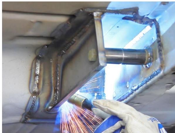
Figure 10 - Weld Inboard Plate
