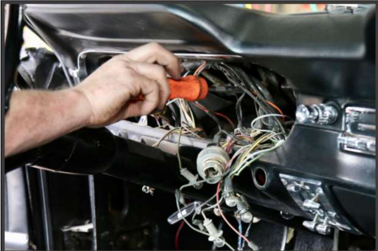
Pretty soon there's a spaghetti bowl of wires secured by a ground connection on a dash brace.
