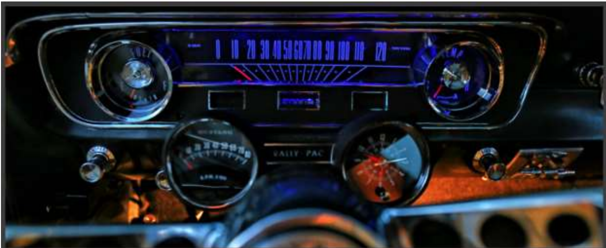
The final step was to install the Rally Pac cluster and to see the fruits of our labor, all lit up. The looks are great, but knowing that fresh wiring had replaced the old, brittle original equipment is the better part of this swap.
