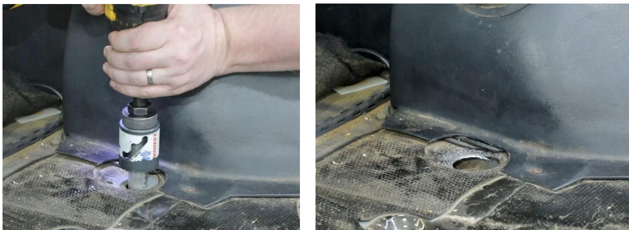
Figure 8 - Drill Access Hole
