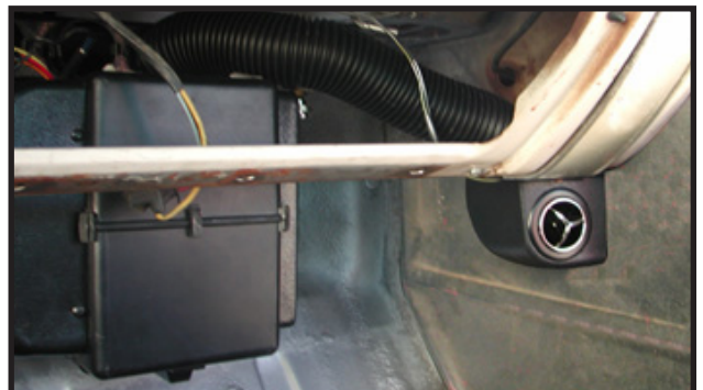
Photo 18 - Install Vent & Duct Hose
