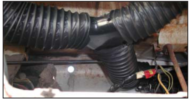
Photo 14 - Connect Defrost Outlets
