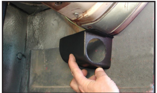
Photo 17 - Install Louver Housing
