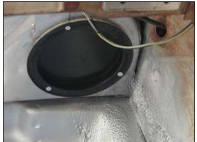
Photo 1 - Install Fresh Air Block-off
