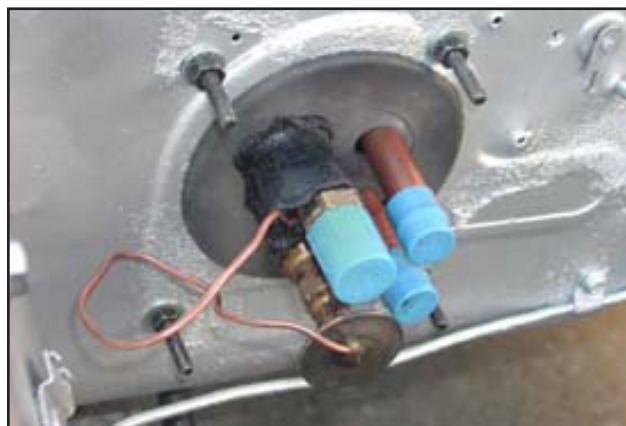
Photo 9 - Wrap Sensor Tube
