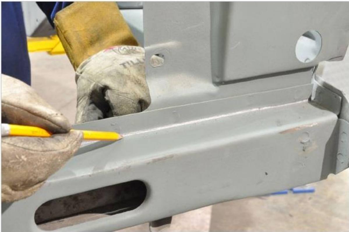
11. Several measurements are taken and the frame marked in various places prior to cutting.
