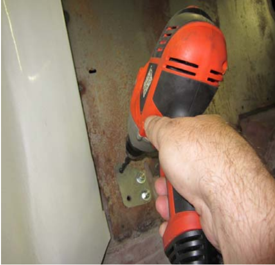
Figure 9. Reinforcement plates inside the car.
