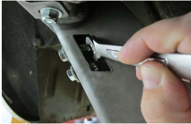
Figure 20. Use access window in Panhard bracket to tighten the hidden 3/8" bolts in the Panhard cross member
